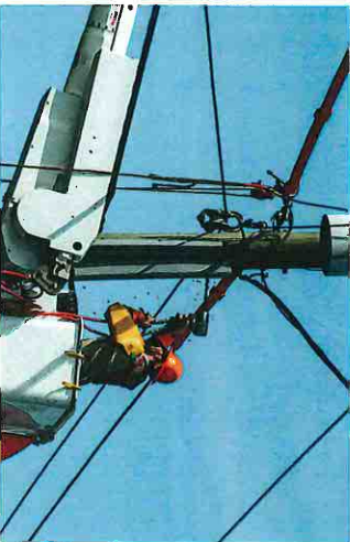
An authorized Dominion Energy contractor installs permanent fiber attachment hardware.
